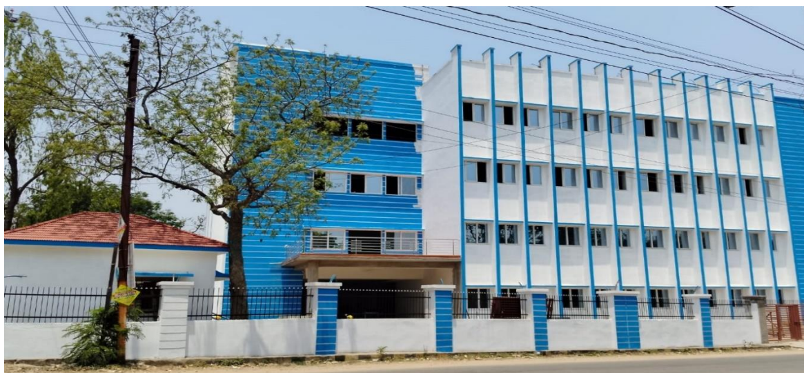
Construction of Commercial office
