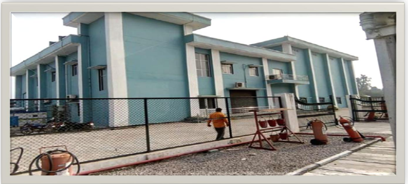
3. Design, Supply, Erection of 132/kV AIS S/s for Bihar State Power Transmission Company Limited
