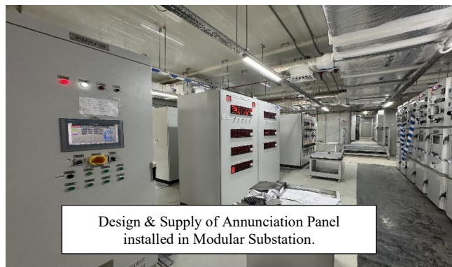
LV Panels and Annunciator Panels
