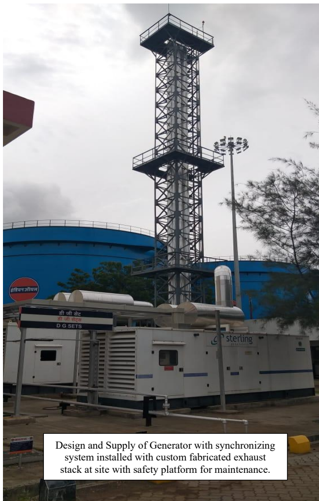
Generator with Exhaust Stack
